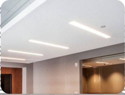
Acoustical drywall ceiling
