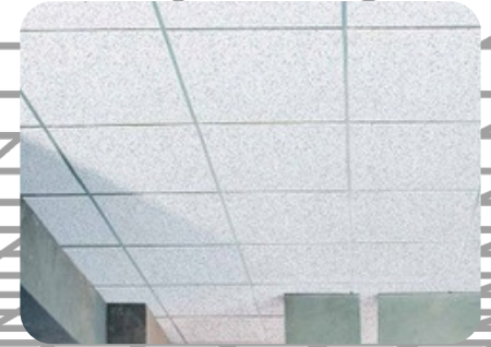
Mineral fiber ceiling
